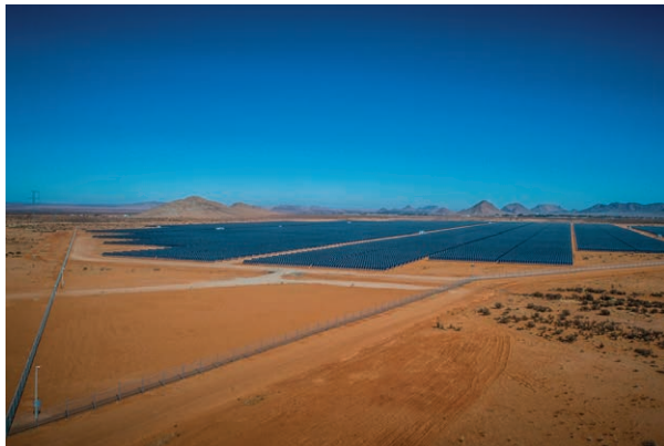
Aggeneys solar farm
